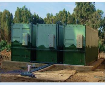
The is a biological treatment as the SBR (Sequencing Biological Reactor), adapted for a capacity from 250 to 5000 IE.
